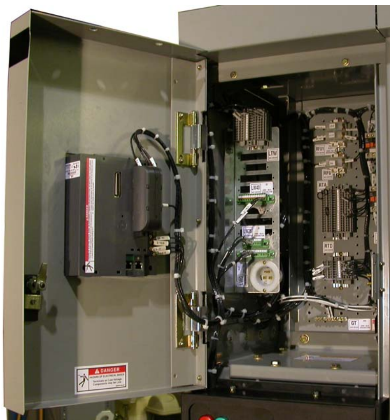
Figure 11: Low-Voltage Components Mounted to the Relay Panel
